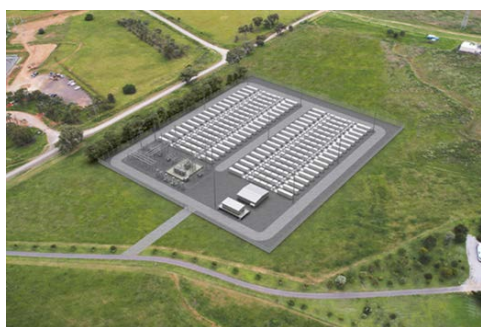
Figure 1.1 Example of a BESS development
