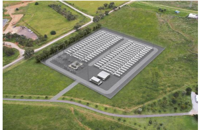
Figure 1.1 Example of a BESS development
